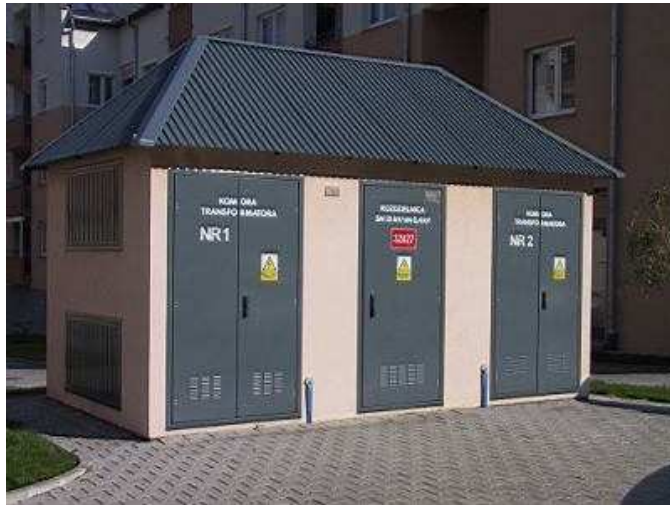
Fig. 6.2. Transformer container station in concrete case type MRw-b (6,1 x 3) 20/2 x 630 [104]
