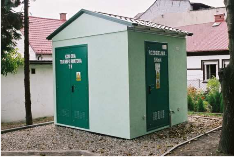
Fig. 6.1. Transformer container station in concrete case type MRw-b1 20/630 [2]
