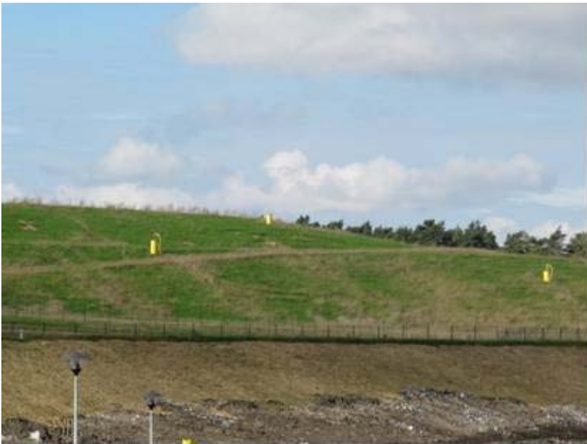
Figure 10-6. Gas collection wells (active collection)
