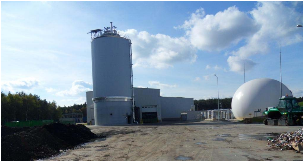
Figure 7-16. A view of a Dranco digestion plant
