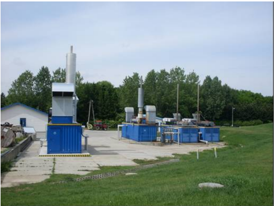
Figure 10-7. CHP units at the landfill site Barycz
