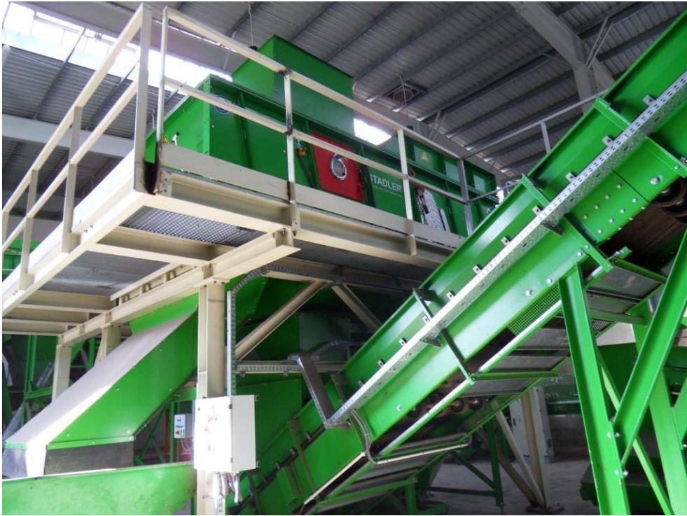
Figure 7-15. Ballistic separator in a Dranco anaerobic digestion plant
