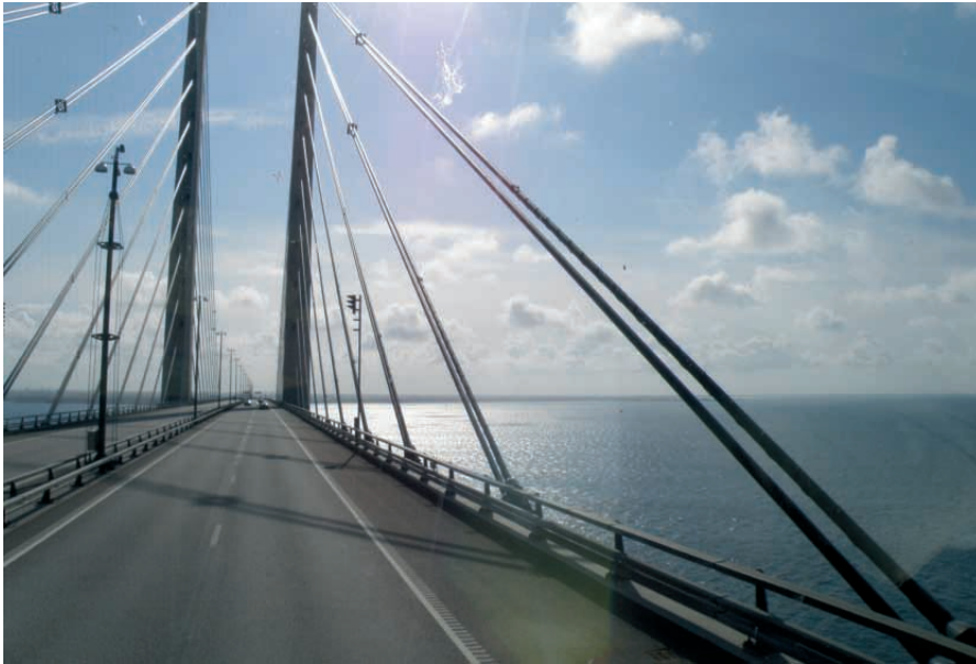
Fig. 1. Bridge over the Sund strait
