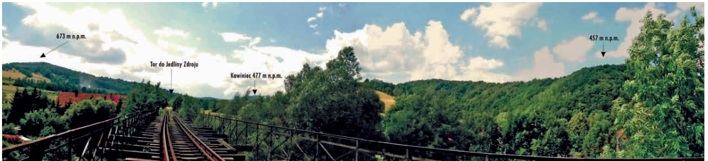
Fig. 11. View from the Jugowice viaduct in the south – western direction, 74,746 km on the route (photo E. Podgórska, 2008)
