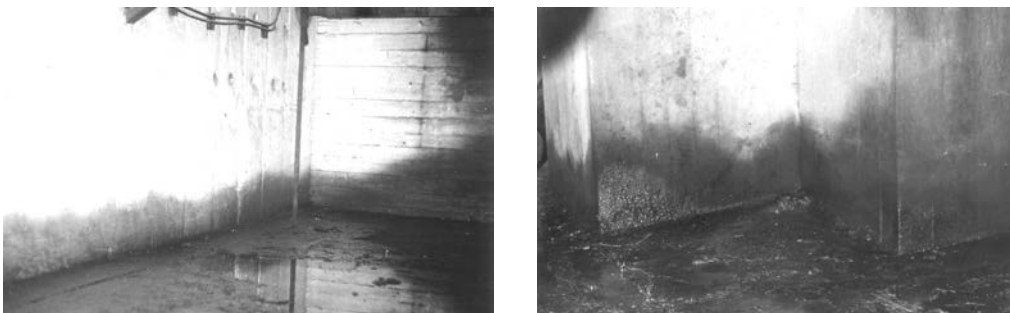
Fig. 4. The lower level of 200 MW turbine foundation
