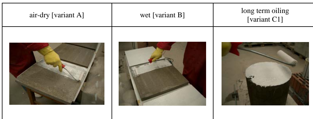
Fig. 6. Spreading of bond layer on concrete surfaces
