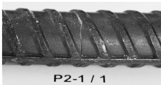
Fig. 3. Fatigue crack in side rebar of beam P2-1
