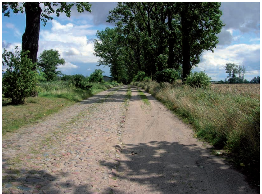
Fig. 1 The road cobbled by field stones with shoulder near Rybitw
