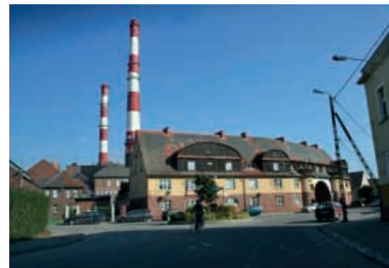
Fig. 14. View of the steelwork in Siechnice
