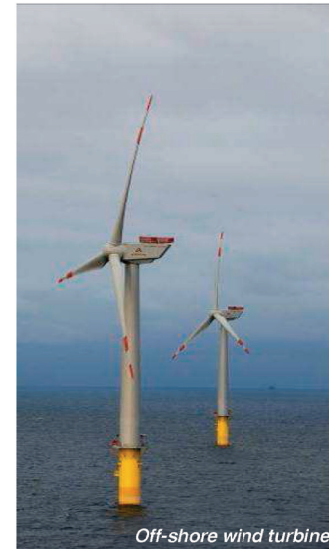
Off-shore wind turbine
