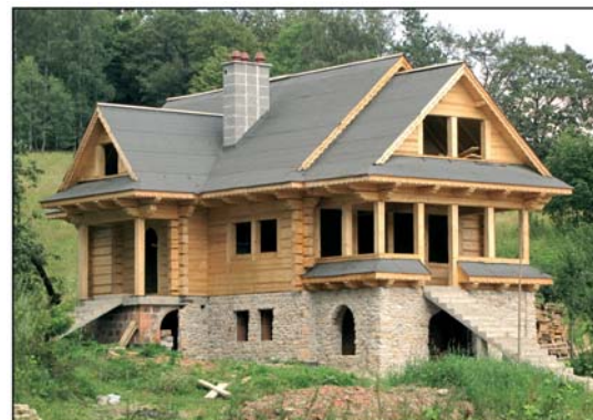
Fig. 3. Weekend Houses representing the building style of the Podhale region – village Orłowice
