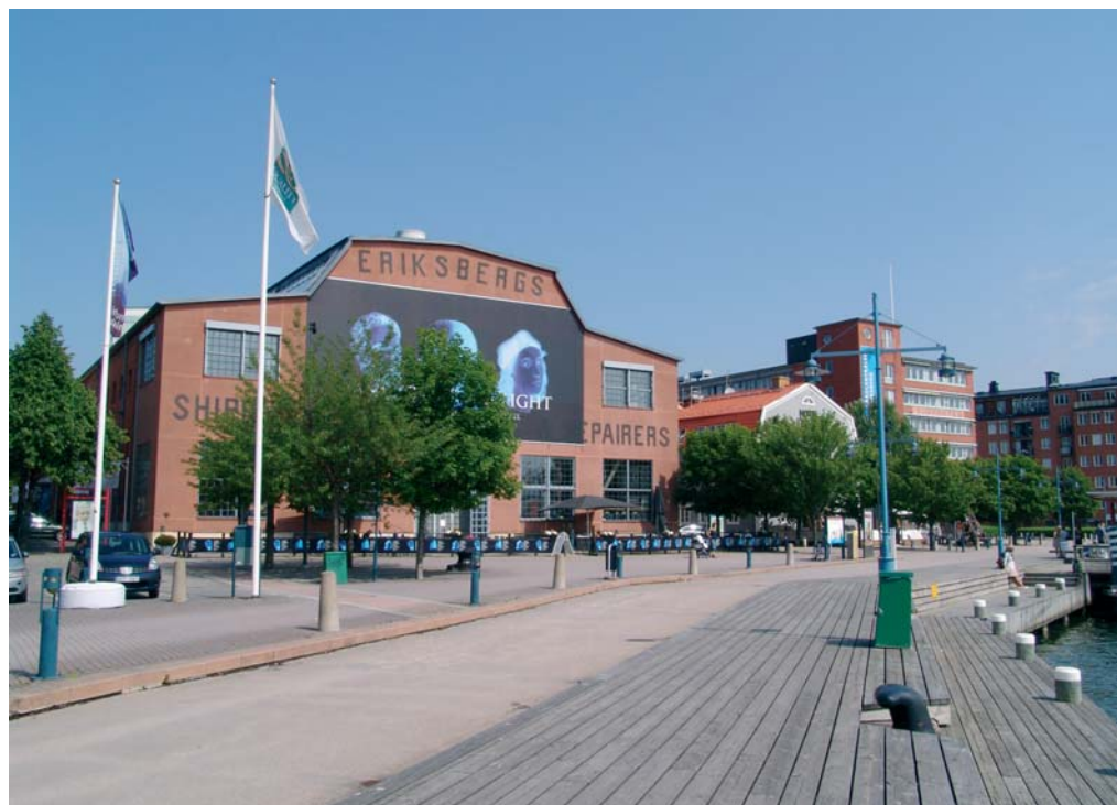
Fig. 6. A node of a public realm network – square within a quay promenade, arranged in front of former shipyard workshops, preserved and adapted for public uses
