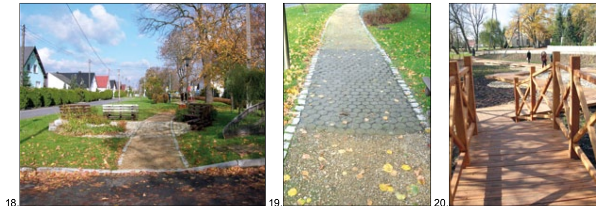
Figures 18–20: The village of Stare Siołkowice in the Opole region in the south-western Poland: (Figure 18) The combination of grass as well as pedestrian stone and sand-like surface in the realized new public space. (Figure 19) The pedestrian path made of gravel and wood next to grass surface. (Figure 20) Wooden pedestrian bridge against the background of gravel and stone surface. Author of the project: WUELS. Source: [19]
