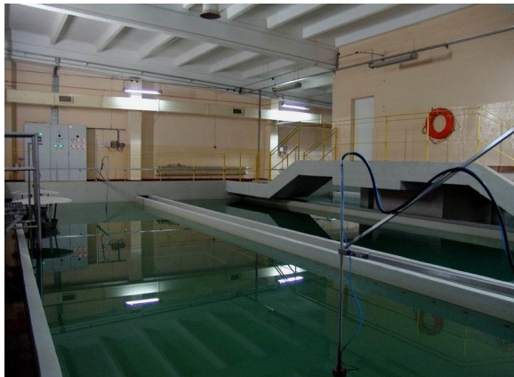
Rys. 2. Pulsator w SUW Pietrasze [13]
