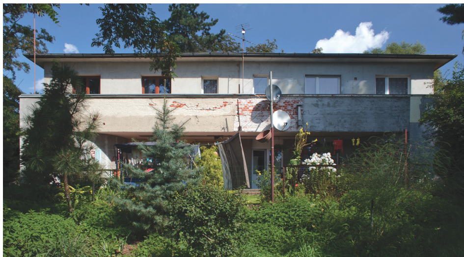
Il. 6. Willa Sterna w Smolcu pod Wrocławiem (fot. B. Bednorz, 2011) Fig. 6. Stern's villa in Smolec (photo by B. Bednorz, 2011)
