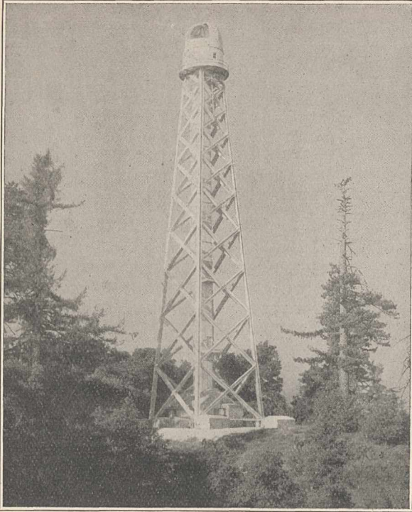
FIG. 8.—The 150-foot tower telescope of the Mount Wilson Observatory. A spectrograph of 75 feet focal length, mounted in a well beneath the base of the tower, is used daily to determine the magnetic polarity and field-strength of all sun-spots seen on the 16.5-inch solar image.
