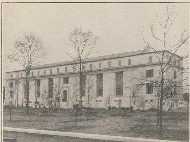
FIG. 1.—New building of the U.S. National Academy of Sciences and National Research Council.
