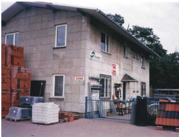
Phot. 1.2. Examples of buildings with walls constructed of gypsum hollow bricks of SOVA type: a) a building of printing house Wrocław, Różana Street; b) apartment building, insulatet with foamed polystyrene + plaster thermic isolation, Wrocław Bielany; c) office-shop building Wrocław Bielany. Phot. S. Klin
