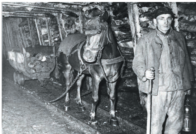
Ryc. 4. Transport materiałów do przodka (Gisman, 1950)
