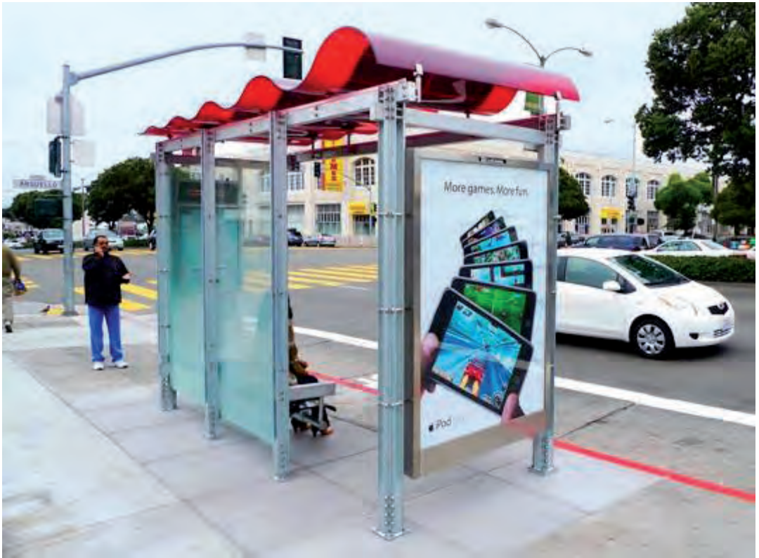
Fig. 7. San Francisco Bus Transit empowered by organic solar cells (by Ryan Hughes, Lundberg Design). [21]
