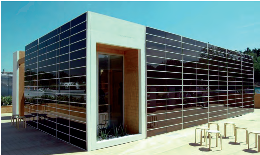
Fig. 6. The Spanish Pavilion at Venice Biennale 2010 equipped with a PV façade (by onyxgreenbuilding.wordpress.com). [20]
