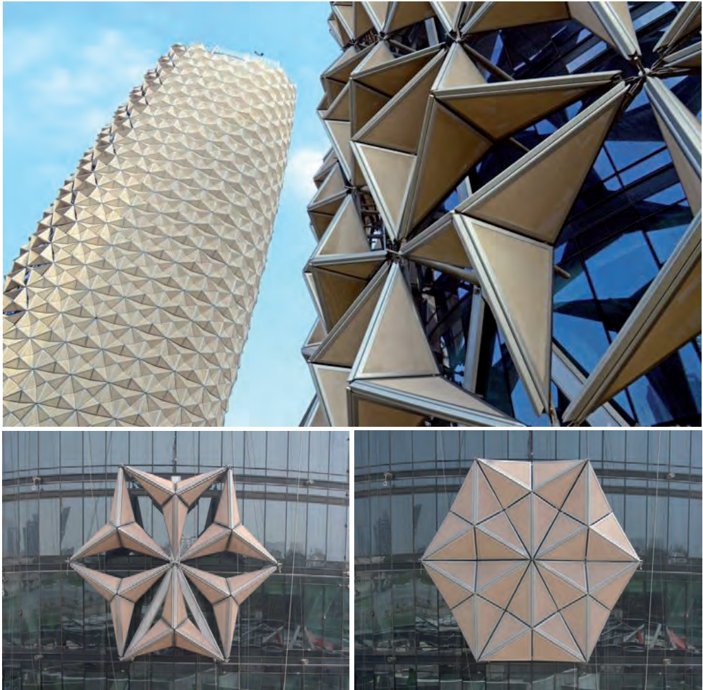
Fig. 1. Bio-inspired architecture - movable elevation of the building operates in analogy to the human pupil, but does not use the same processes (by Aedas Architecture). [7]
