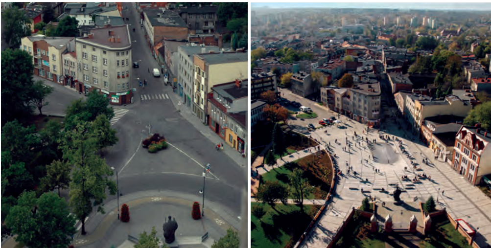
Fig. 5. The comparison between previous (left) and current (right) state of Plac Wodny.
