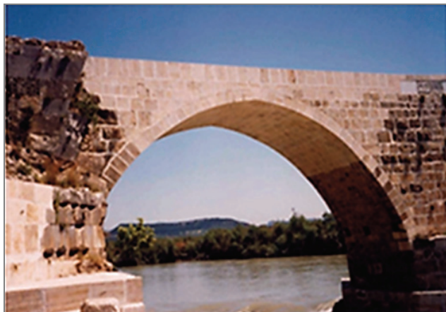
Fig. 1. Present-day use of travertine in the renovation of historical engineering objects – Belkis bridge (Turkey) (photo by J. Pinińska)
