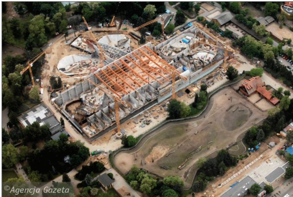
Fig. 4a. Foundation slab of the “Africa Pavilion” complex (photo from [17])
