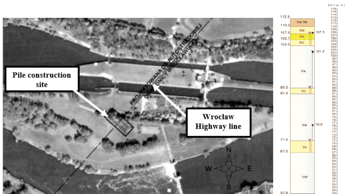
Fig. 2. Construction site and soil profile [2]
