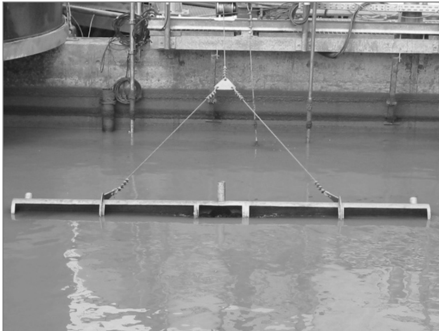
Fig. 1. Photo of decanter during decanting at the Gemüse Meyer works
