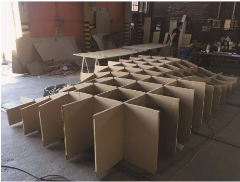
Figure 4. Roof assembling, photo by J. Łątka
