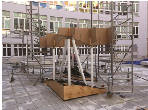
Figure 5. Under construction, photo by J. Łątka
