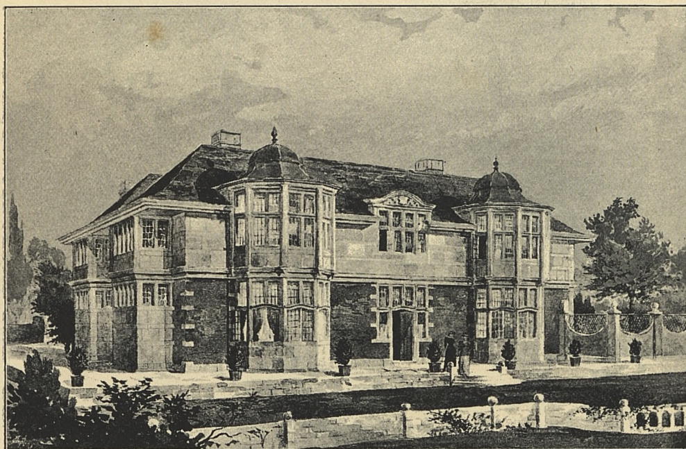
House at Winchfield, Hants, for Capt. F. Young, FAIRFAX B. WADE, F.R.I.B.A., Architect. (For Plans, see p. 142.)
