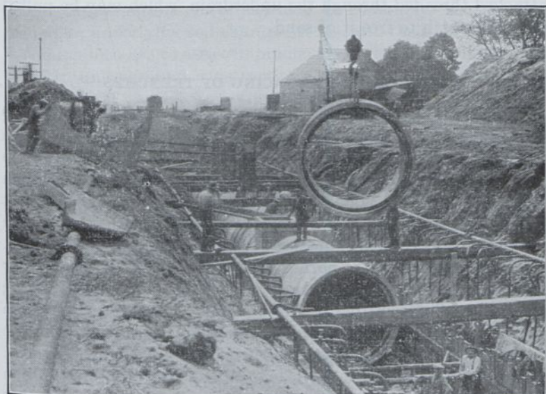
FIG. 115.—Sewer trench unwatered by well-points and pumps.
