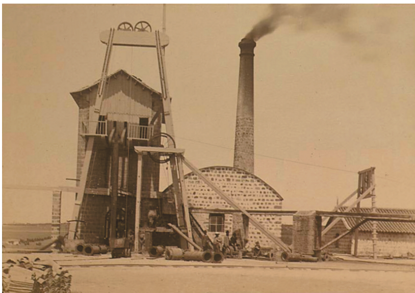
Fig. 2. La Tortilla Mine, the 60inch Cornish beam engine on Palmerston Shaft (National Archives, Madrid, ES.28079.AHN/4.2.13)
