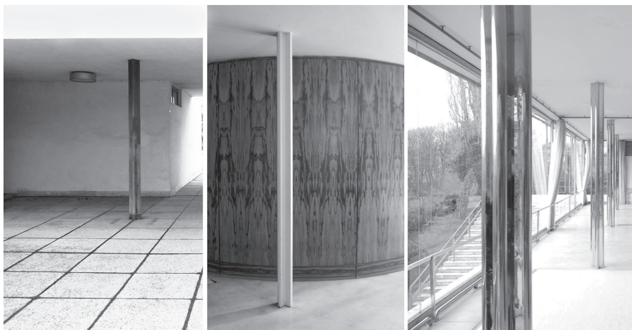
Fig. 7. The three types of columns in Villa Tugendhat (photo by A. Cervilla García, December 2009)
