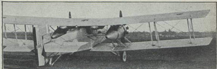
Boulton-Paul „Bugle I“ (1924) Kbn 3; E: J. D. North b = 19,10 m; l = 12,10 m; T = 86,00 m 2 ; L = 2,20 t; N = 1,56 t; G = 3,76 t; V = 83–200 km/h; H = 5,0 km; M: 2 × Bristol 420 PS-HP-CV = 840 PS-HP-CV; Bst.: S, St.
