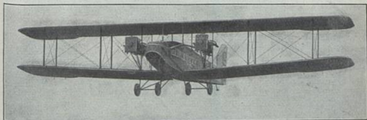
Handley Page W 10 (1925) V 16; E: F. Handley Page b = 22,86 m; l = 18,08 m; T = 137,7 m 2 ; L = 3,88 t; N = 2,36 t; G = 6,25 t; V = 89—174 km/h; H = 3,3 km; St = 0,21 km/1'; M: 2 × Napier 450 PS-HP-CV = 900 PS-HP-CV; Bst.: H, St, S.
