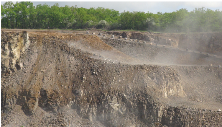
Fig. 2. Excavation in the Męcinka mine (author's photo)
