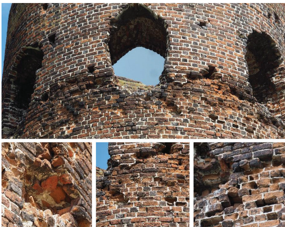
Fig. 8. Castle in Koło. Examples of the state of preservation of the tower walls (photo by K. Polak, 2020)
