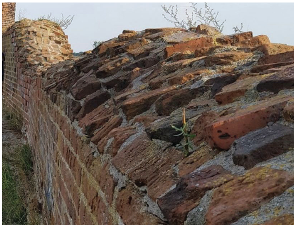
Fig. 9. Castle in Koło. The crown of the breastwork softly prepared during renovation works in the 20 th century (photo by K. Witkowska, 2020)
