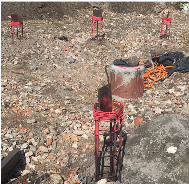
Figure 4: Part of the site prepared for static load testing (image captured by the author).
