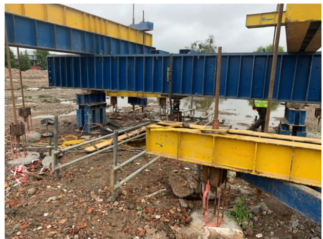
Figure 6: Completed static load test site ready for testing (image obtained from authors' library).
