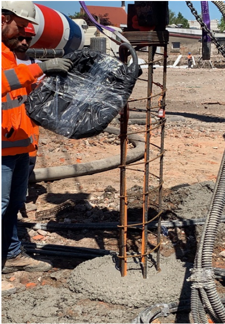
Figure 3: Pile designed for testing with visible extensometers attached to the reinforcing steel while casting (image captured by the author).
