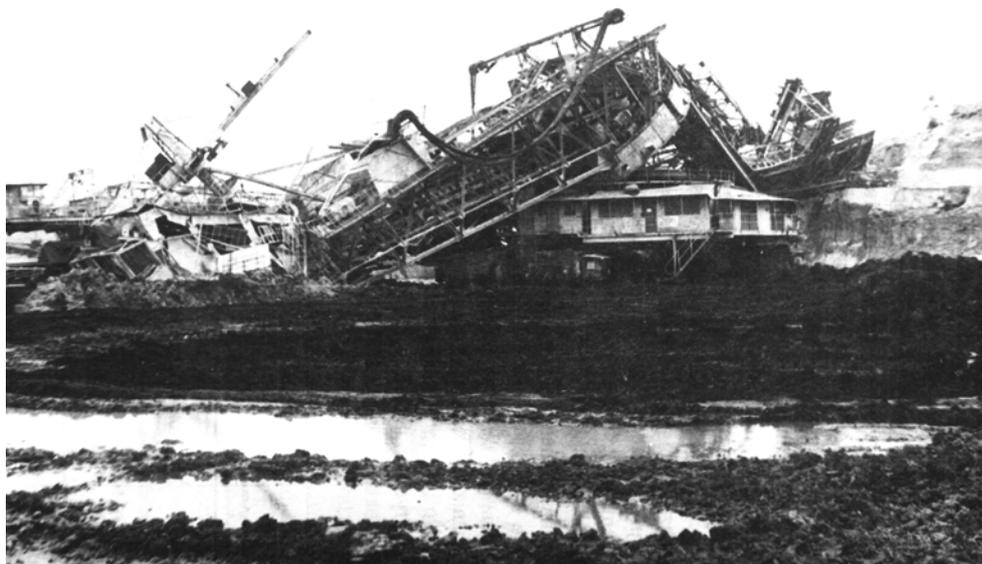
Fig. 1.2. Failure of SchRs1200 bucket wheel excavator [1.1].
