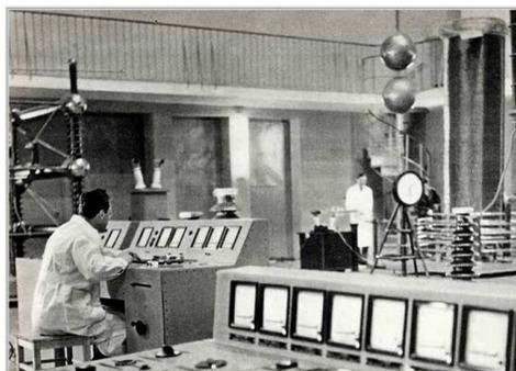
**Fig. 4. Van der Graaff's generator (on the left) and Tesla transformer (on the right) in the third HV laboratory (picture from 1960s)**
