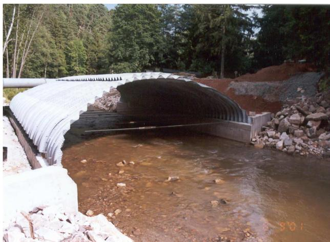
Fig. 2. Headwater side view of assembled steel shell structure before backfilling (test stage I)
