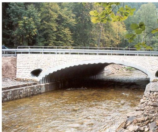
Fig. 6. Headwater side view of steel road bridge made from *Super Cor* corrugated plates located in Polanica Zdrój
