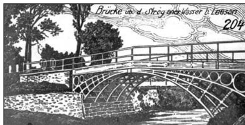
Fig. 4. Slender and flat structure of the Łazany bridge (compare to Figure 3) [7]
