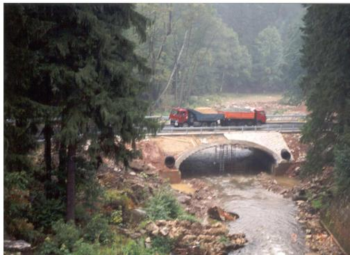
Fig. 3. Top view of bridge during tests under load scheme II in test stage II
