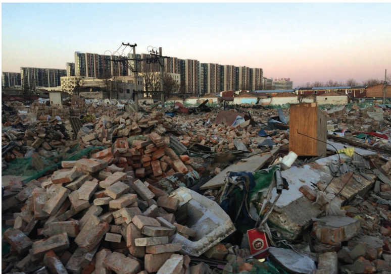
Fig. 4. Sanyingmen neighbourhood after demolition (photograph: Tom Phillips)
